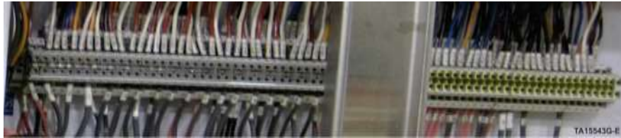
Figure 8. Terminal strip TS1
