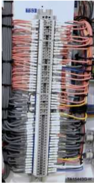
Figure 11. Terminal strip TS3
